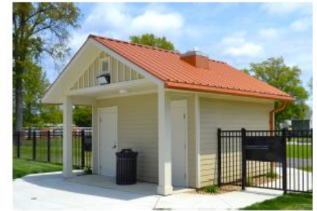
RESTROOM EXAMPLE: ELYRIA, OH
