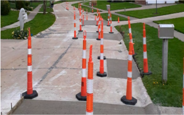
Concrete Repairs Underway
