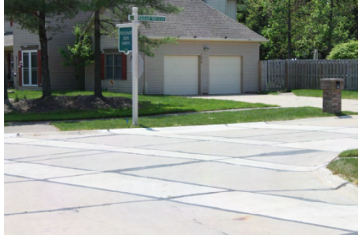
Completed Concrete Repair
