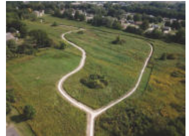
North Park— Completed Trail
