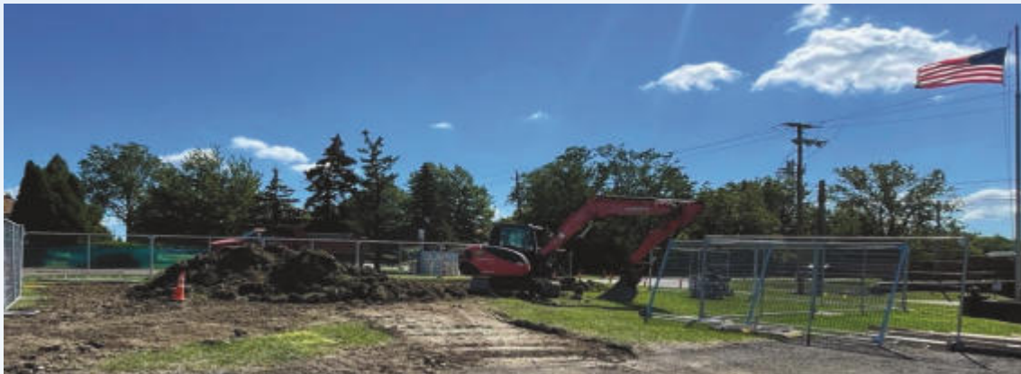
Construction on new Community Gazebo
