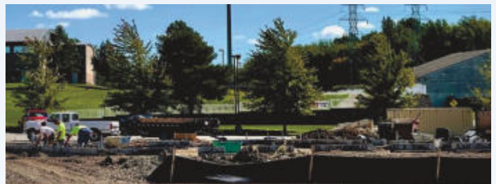
Construction has begun on the new Dairy Queen
